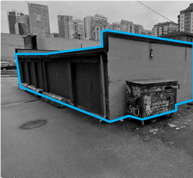
Image : Poor treatment of corner blocks with blank facades results in unsafe nooks.
