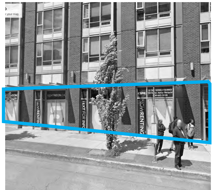
Image : Avoid large expanses of frontage without pedestrian entry along the main street.
