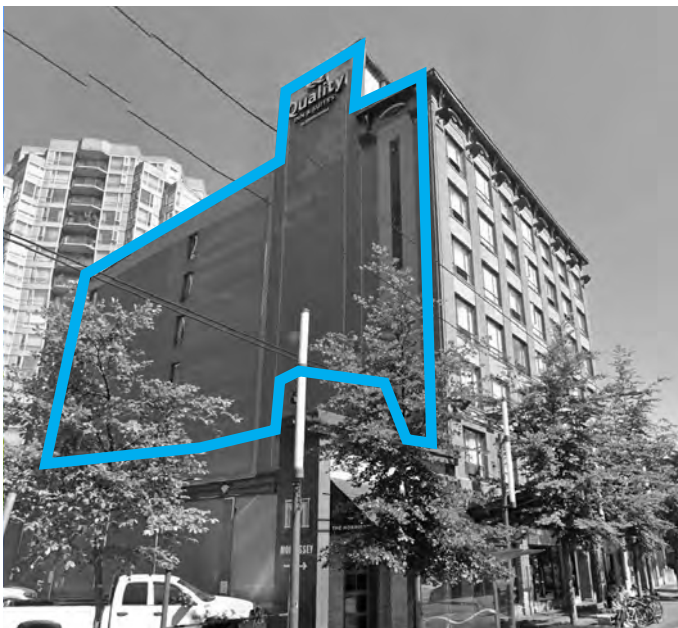
Image : Blank walls to be avoided, either openings via balconies or set backs in the massing.
