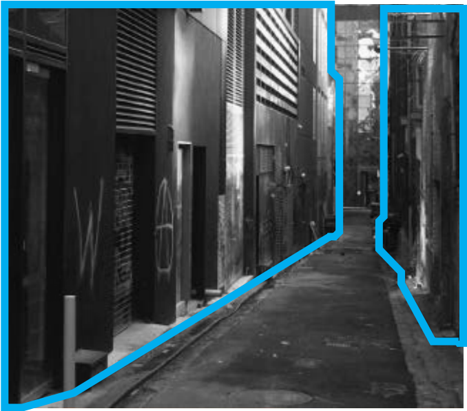
Image: Dead rear elevation that discourages laneway activation.
