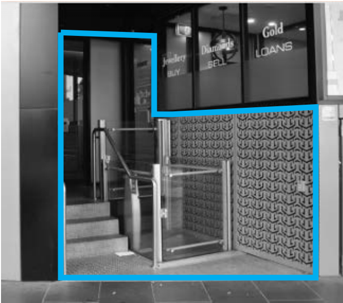
Image: Platforms and lifts to be avoided where they gather unsafe spaces.
